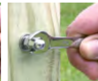
Cut thread leaving 1/4” and install acorn nut
