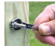
Tighten nut to tension
