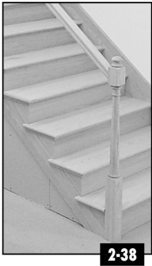
STARTING NEWELS A 5" top block will always work at the beginning of the stair. Larger top blocks are unnecessary and can appear top-heavy. PHOTO 2-38.
