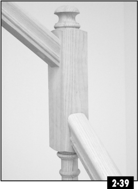
INTERMEDIATE LANDING NEWELS Intermediate landing newels will have angled rail entering and exiting the upper square block from adjacent sides. Because the newel is basically making up for two rise dimensions in the stair ( the last rise before the intermediate landing as well as the first rise of the second straight run ), a longer square block is necessary to keep consistent rake rail heights from the first run to the second. A newel with a minimum 13" top block will be required. PHOTO 2-39.
