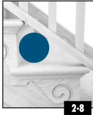
A related "sphere code" relates to a stair that uses shoe rail (See Photo 2-74) on an open stair. The size of the triangle formed by the tread, riser, and the bottom of the shoe rail is also governed by a sphere size, usually 6". PHOTO 2-8.
