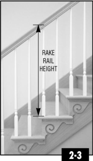
RAKE RAIL HEIGHT Rake rail heights are measured from top of the leading edge of the nosing to the point at the top of the rail directly above. PHOTO 2-3.
