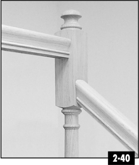
BALCONY LANDING NEWELS Balcony newels will have angled rail entering from the lower side of the newel with level rail exiting from the top of the upper block. Because only one rise dimension is involved, a 10" top block will normally be required. PHOTO 2-40.
