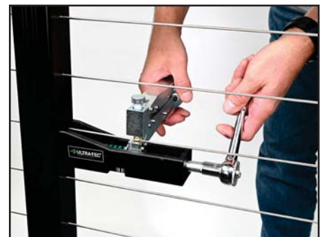
Rotate using ratchet to pull tension
