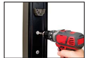
Fasten Threaded Connectors
