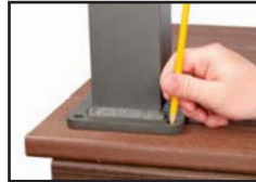
Mark and Pre-drill Holes
